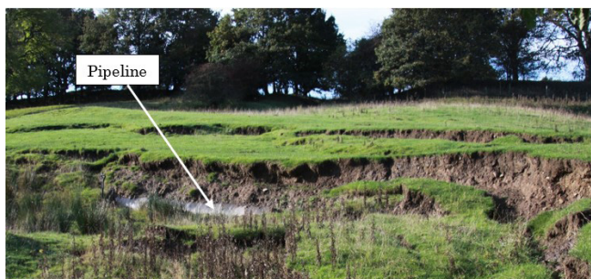
Figure 2. Landslides may affect pipeline integrity, making monitoring or stresses essential.
